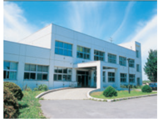
管理棟 Administration Building, Fujisaki Farm ①
